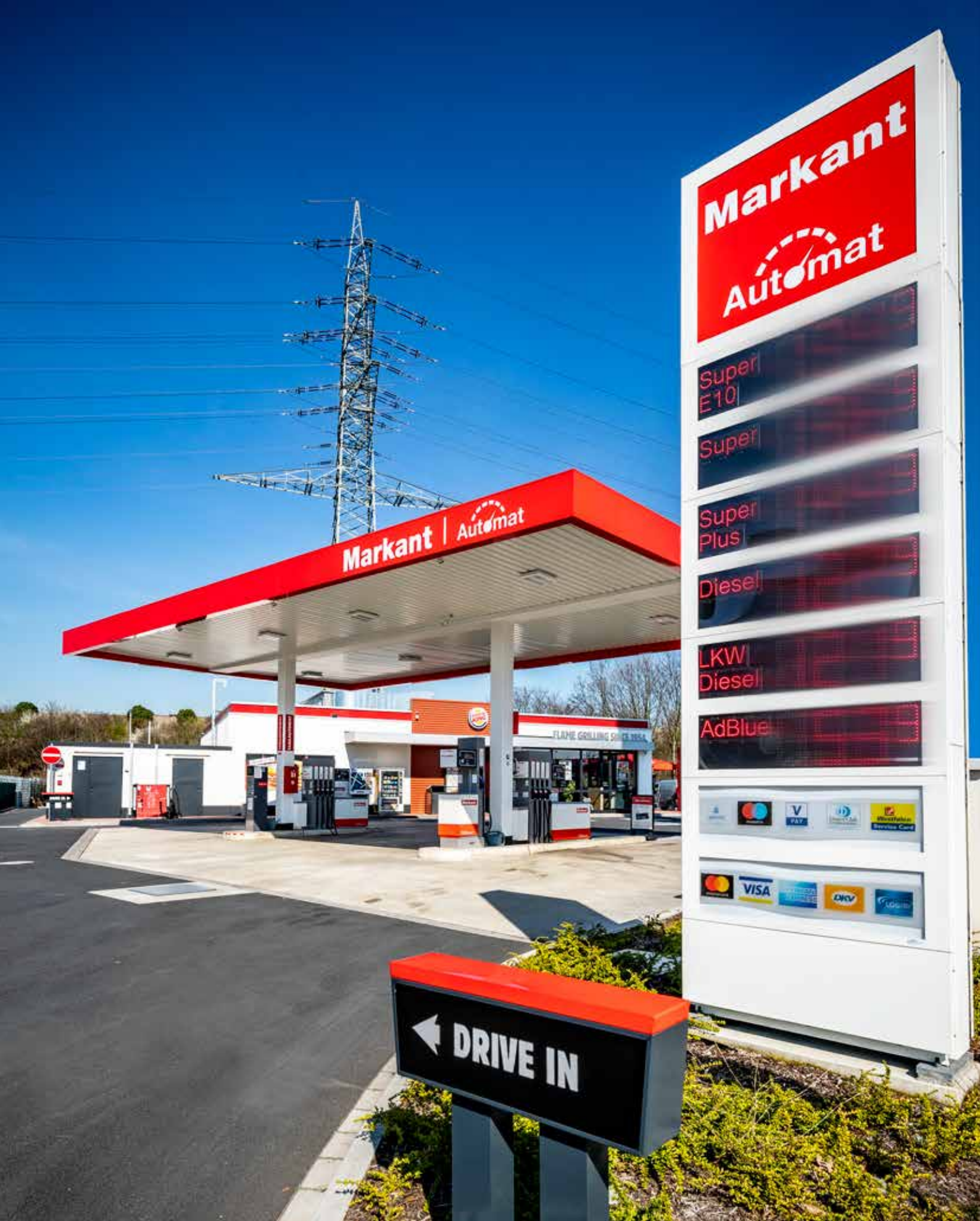
A refuel followed by a Burger King: the new unmanned service station in Düsseldorf-Reisholz.
