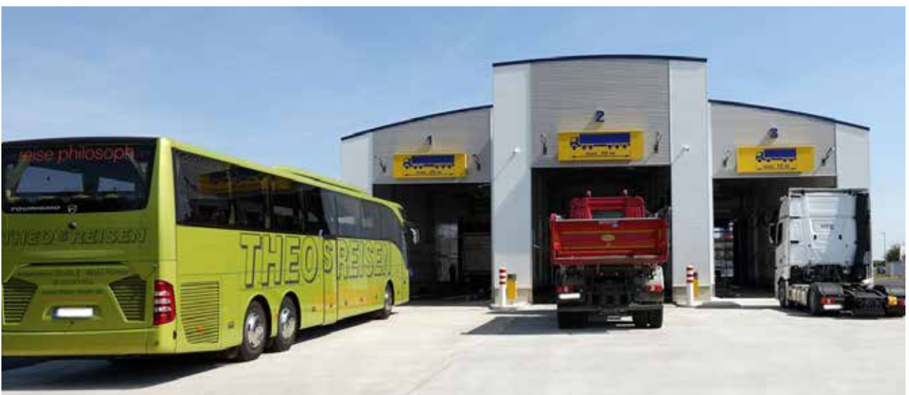
Truck Wash Amelsbüren can clean up to nine trucks, buses or caravans per hour.
