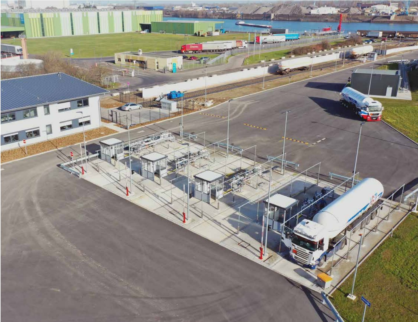
The Krefeld depot went into pilot operation at the beginning of 2021.
