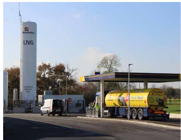
On 18 November, the first stationary LNG service station in the Münster area went into operation at the Westfalen service station in Münster-Amelsbüren.
