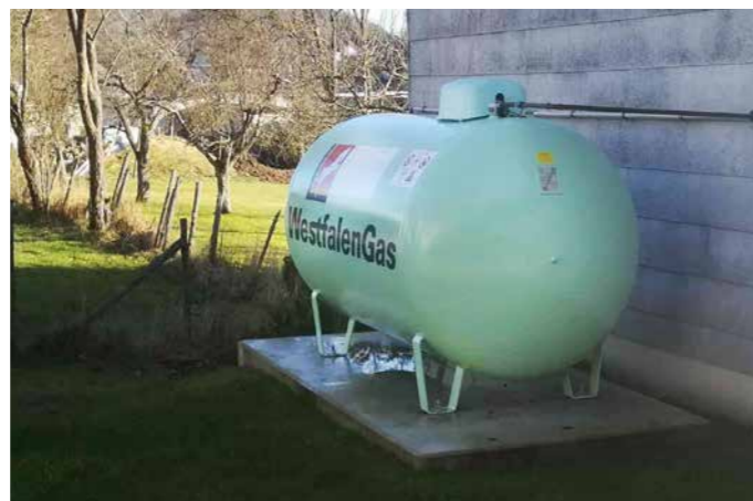
Quick help: a newly installed Westfalengas tank in the flooded region.
