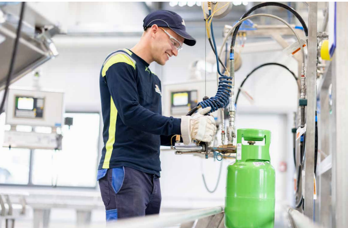
New, ergonomically optimized refrigerant filling facility in Münster-Gelmer.
